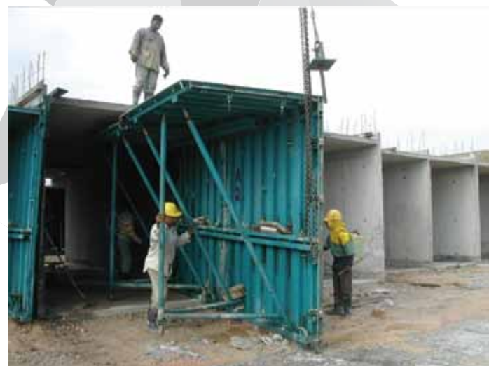
Innovative method of Tunnel Form
