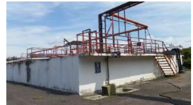
Figure 1: Collection of POME final discharge.
