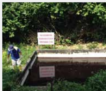
Figure 1. Final discharge pond in palm oil mill
