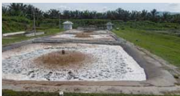
Figure 1. POME treatment system in palm oil mill. (Aerobic pond)
